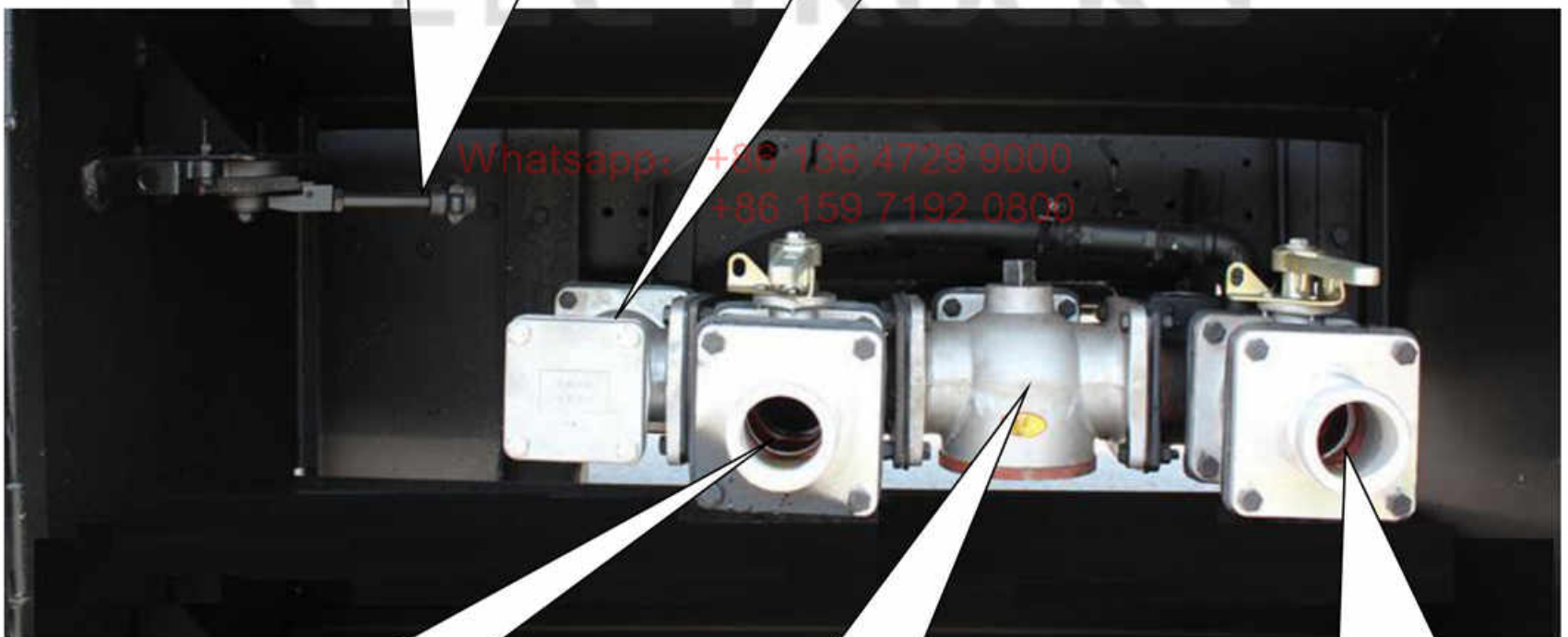
Fuel Inlet Valve (Entrance) Pumping fuel into the tank
